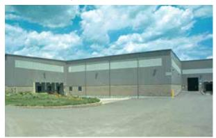
Wallite panels are engineered with an advanced polymer system for premium weathering and exceptional color stability – providing up to ten times better performance than conventional FRP panels. Wallites will not rust, mold, mildew or corrode. Wallites are white translucent panels available in Panel Rib or Vee Rib profiles. With a nominal 3'-0" wide coverage, the standard Wallite length is 5'-4". Custom lengths are available with minimum run requirements.
